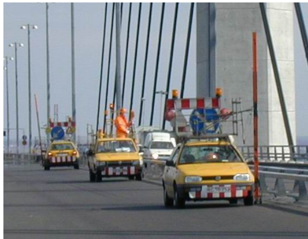
figure 3.1: Motorized leveling on the High Bridge
